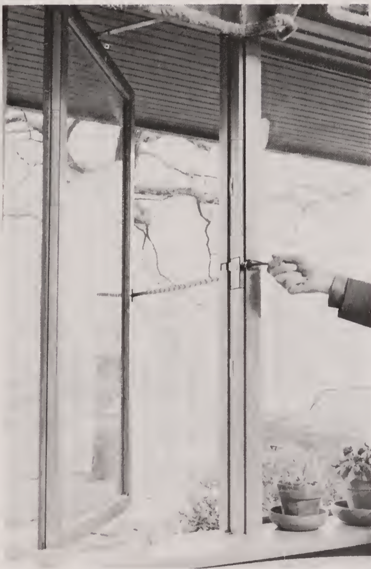
Both sides of the glass can be washed from the inside when casement windows are hinged this way.
